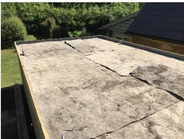
Filter layer of geotextile
